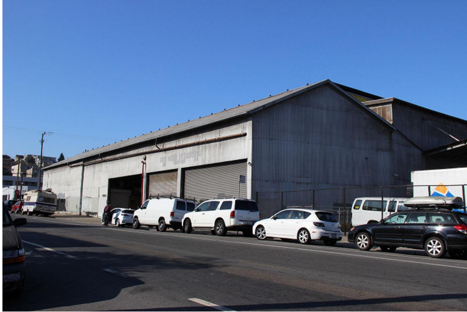
Figure 12. Warehouse at 1100 17 th Street, looking southwest, 2014 Source: Christopher VerPlanck
