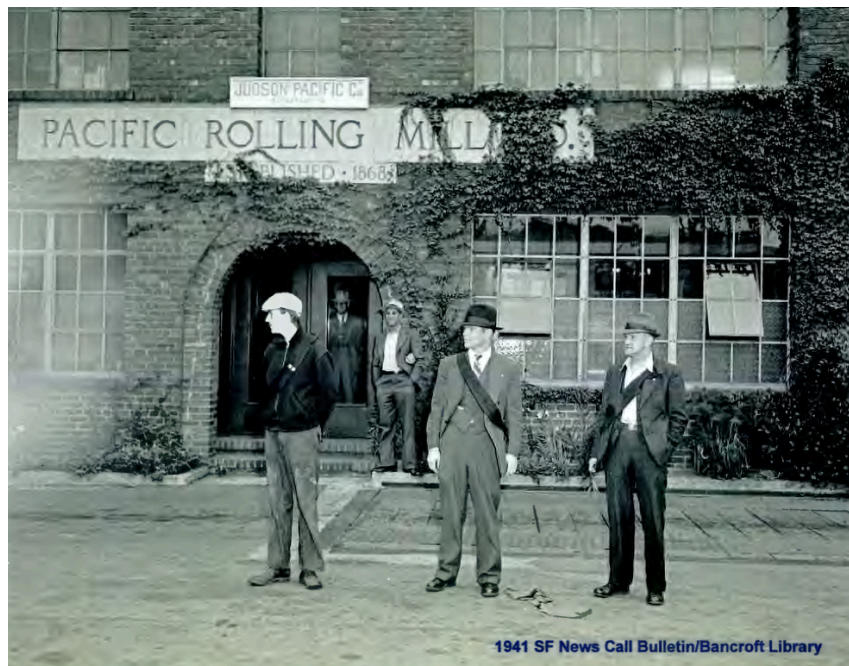
Figure 1: Three men stand alongside a grade-level truck scale in front of the Judson-Pacific Co. building at 1200 17 th Street. Extant building features include: the brick facade, sills, and arched portal; multi-light steel sash windows; and cast-cement sign. The sign notes the company's establishment date as 1868. Image dated 1941. Source: Bancroft Library, University of California, Berkeley.
