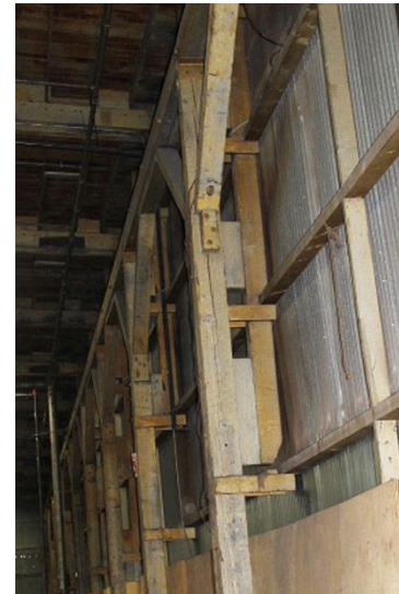
Figure 24. Sistered columns, 2014
