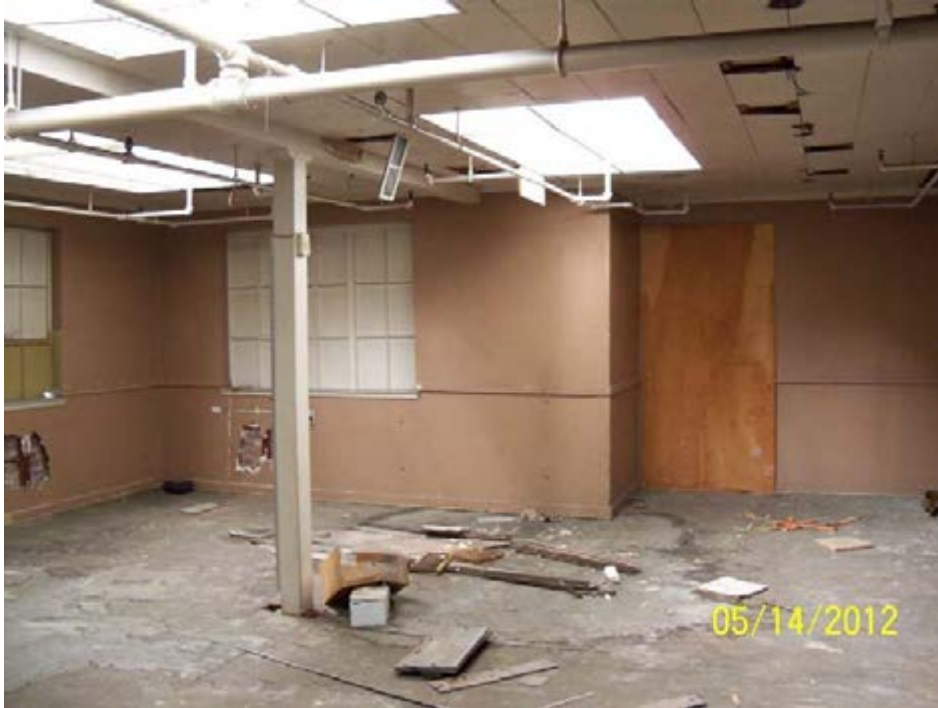
Figure IV.B-8: Interior of Brick Office Building at 1200 17th Street, 2012
