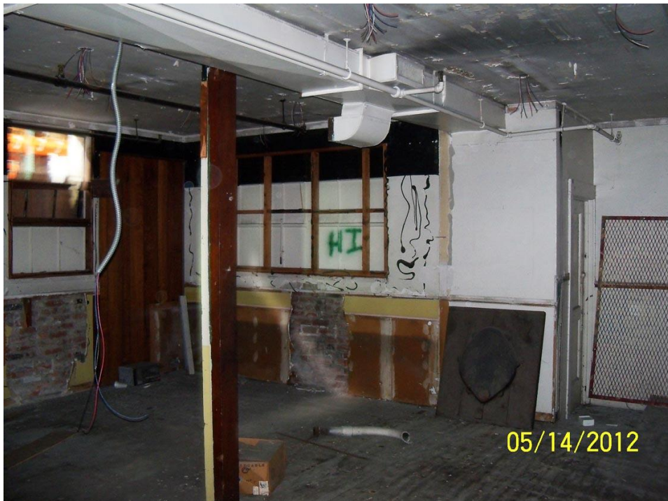
Figure 29. Interior of office building: first floor looking northeast, 2012 Source: Christopher VerPlanck
