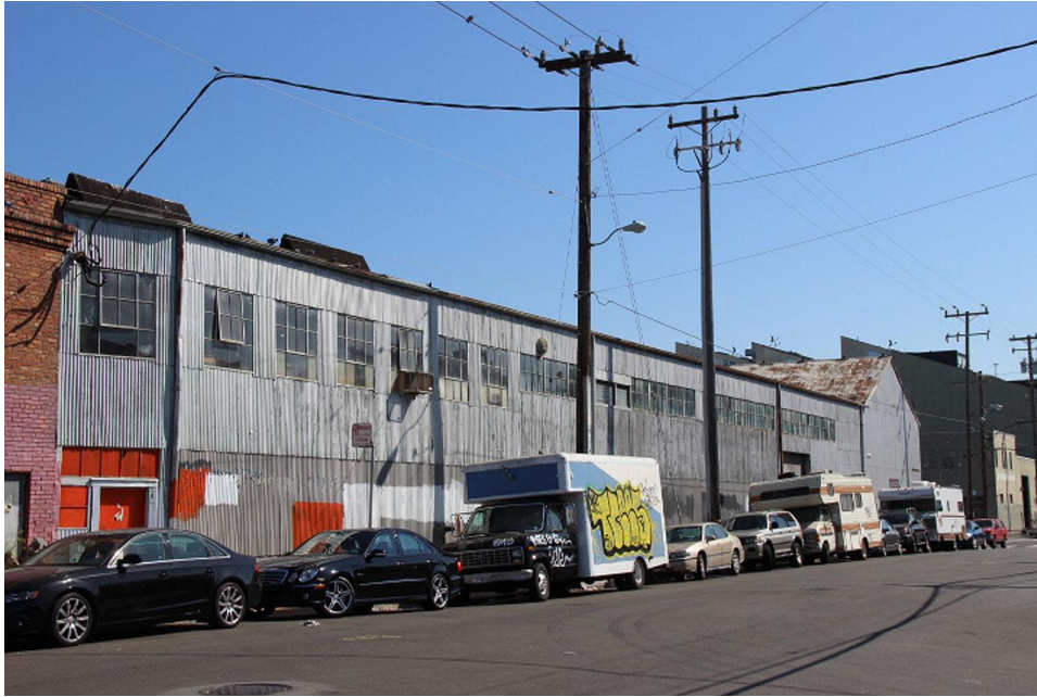
Figure 15. South façade of metal-clad warehouse at 1200 17 th Street, 2014 Source: Christopher VerPlanck
