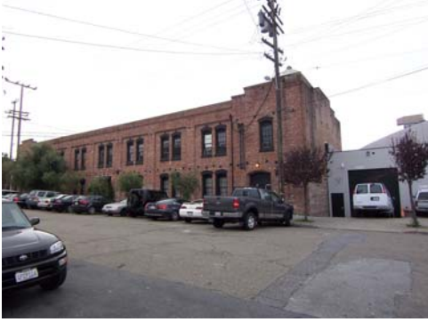
100_5210.JPG, 11/16/2007, view to SW
