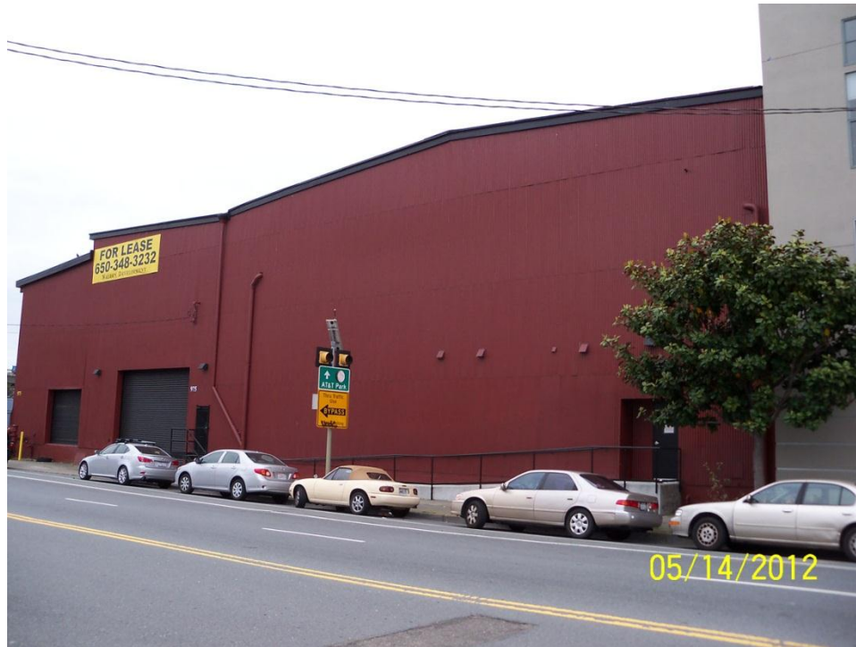
Figure 20. North façade of metal-clad warehouse at 1200 17 th Street, 2012 Source: Christopher VerPlanck
