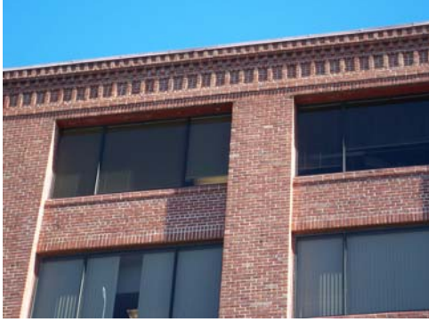
100_5885.JPG, 11/21/07, cornice detail
