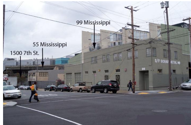
Figure 5. 99 Mississippi Street, looking northeast, 2012 Source: Christopher VerPlanck
