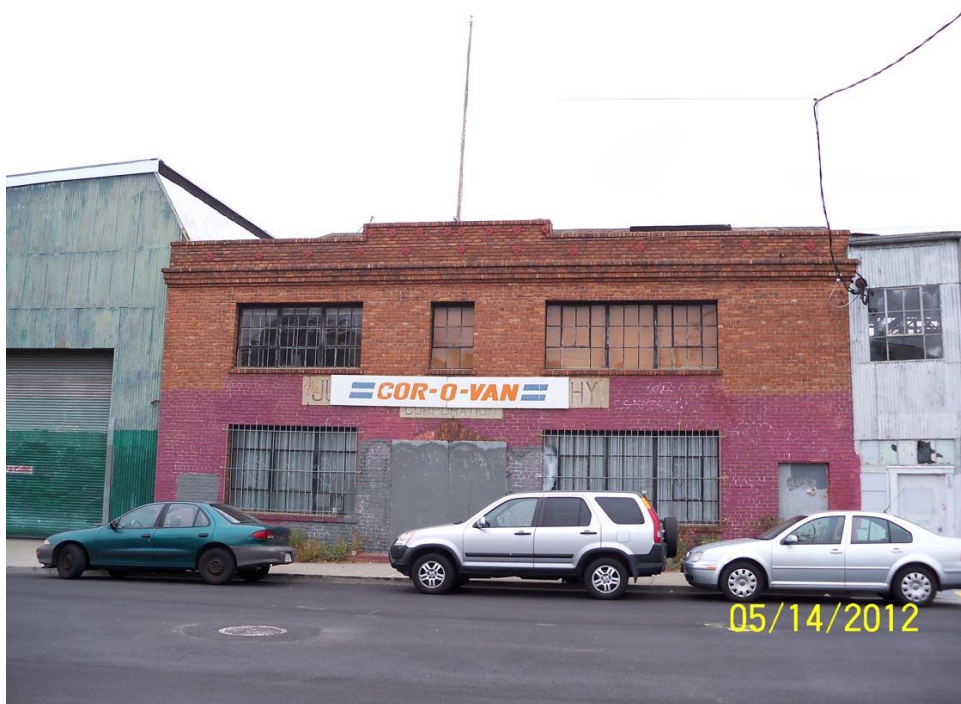
Figure 25. South (primary) façade of 1200 17 th Street, 2012 Source: Christopher VerPlanck
