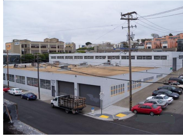
Figure 7. 1111 17 th Street, looking southeast, 2012 Source: Christopher VerPlanck
