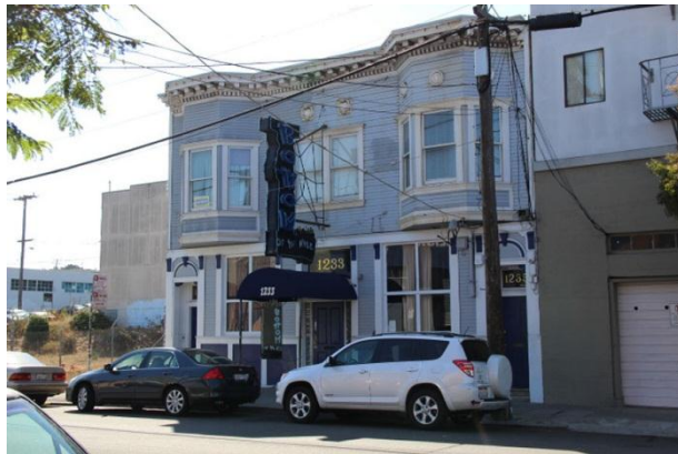
Figure 8. 1231 17 th Street, looking southeast, 2014 Source: Christopher VerPlanck
