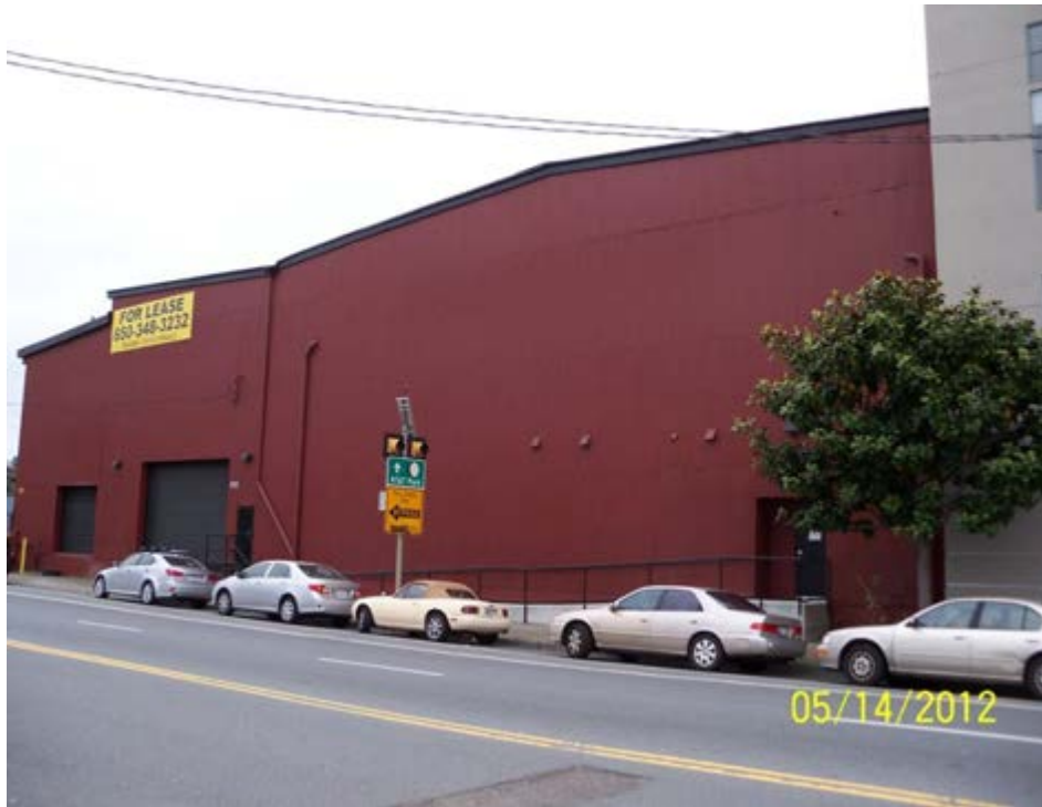
Figure IV.B-6: North Façade of Warehouse at 1210 17th Street/975 16 th Street, looking southeast on 16 th Street, 2012
