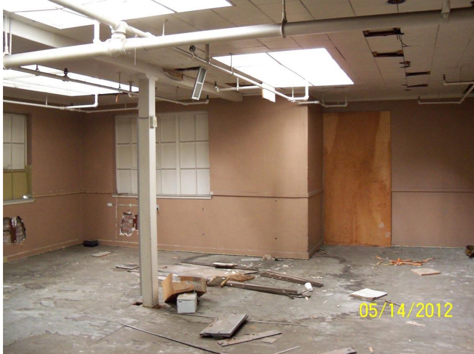
Figure 30. Interior of 1200 17 th Street: second floor looking northeast, 2012 Source: Christopher VerPlanck
