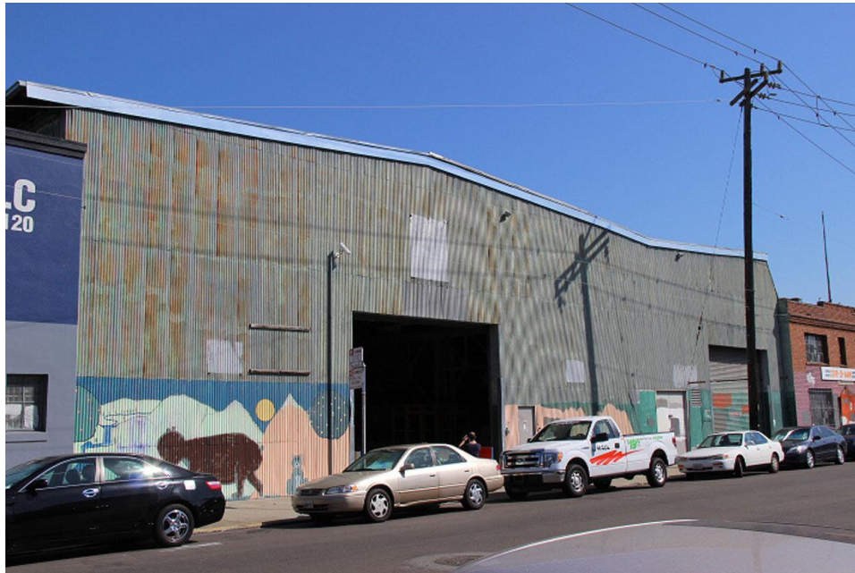
Figure 19. South façade of metal-clad warehouse at 1200 17 th Street, 2014
