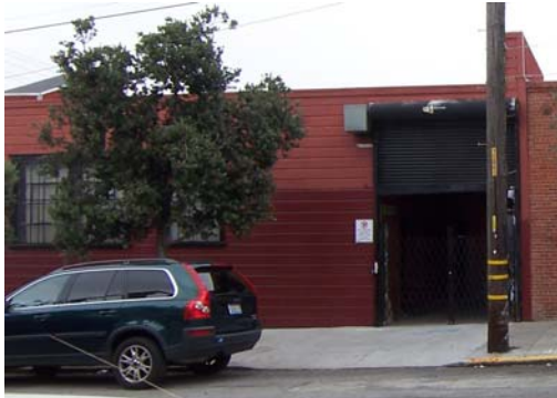
100_5206-1, 11/16/07, view to N, eastern building
