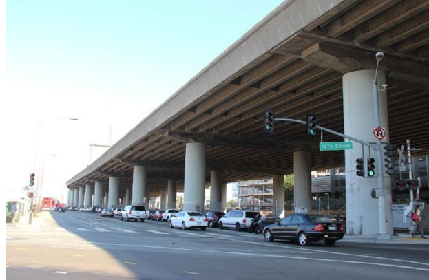
Figure 3. Interstate 280 viaduct, looking northeast, 2014 Source: Christopher VerPlanck
