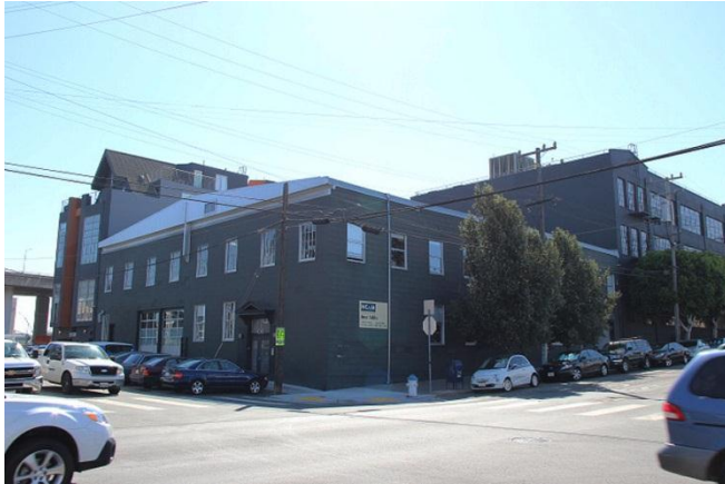
Figure 6. 1045 17 th Street, looking southeast, 2014 Source: Christopher VerPlanck
