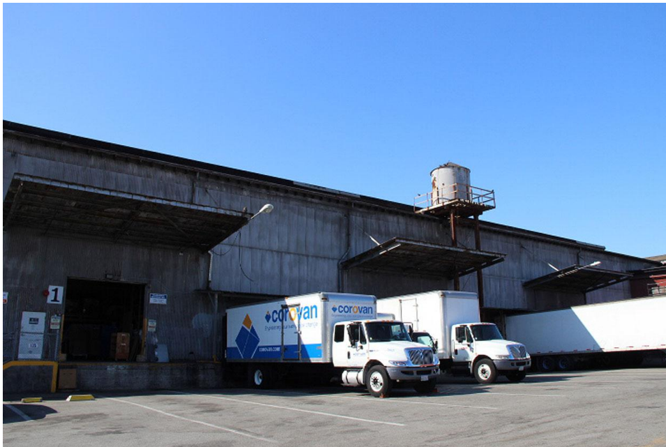
Figure 16. North façade of metal-clad warehouse at 1200 17 th Street, 2014 Source: Christopher VerPlanck
