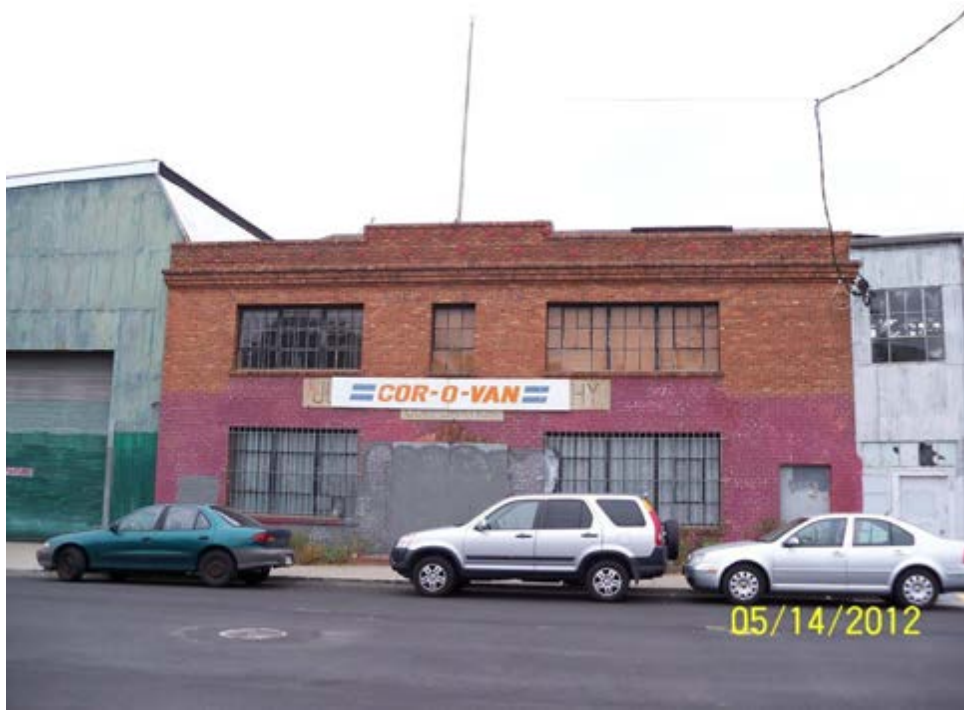
Figure IV.B-7: South Façade of Brick Office Building at 1200 17th Street, looking north on 17 th Street, 2012
