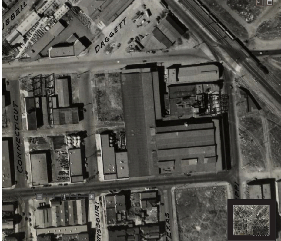
Figure 2: This aerial view shows the Pacific Rolling Mill Co. buildings at 1200 17 th Street at the center of this photograph. The location of the site's extant buildings is unchanged. The original footprint of the site's principal buildings has remained virtually unchanged to the present. Image dated 1938. Source: David Rumsey Map Collection (online).
