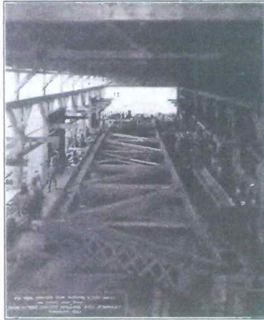
Largest Steel Truss made by Pacific Rolling Mills for Native Sons' Building, San Francisco
