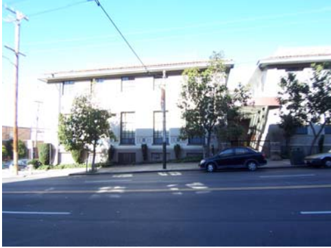
100_6186.JPG, 11/23/07, view to N
