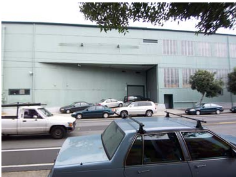
100_5520.JPG, 11/19/2007, west elevation rail car entrance
