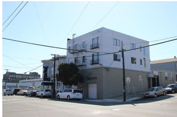
Figure 9. 1239 17 th Street, looking southeast, 2014 Source: Christopher VerPlanck
