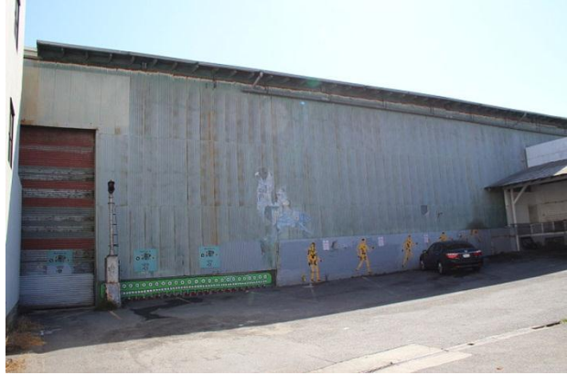
Figure 22. West façade of metal-clad warehouse at 1200 17 th Street, 2014
