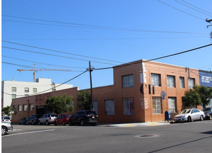
Figure 10. 1250 17 th Street, looking northeast, 2014 Source: Christopher VerPlanck
