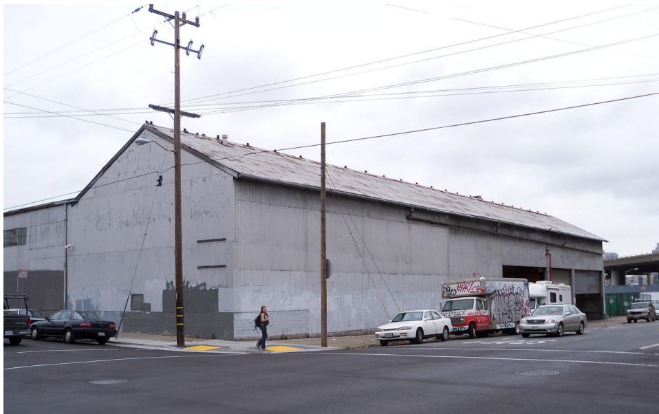
Figure 13. Warehouse at 1100 17 th Street, looking northwest, 2012 Source: Christopher VerPlanck
