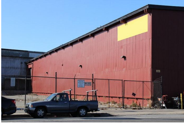
Figure 21. East façade of metal-clad warehouse at 1200 17 th Street, 2014
